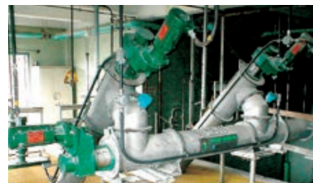
Auger Monsters and cross conveyor
