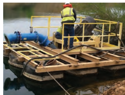
PREPARE THE NEWLY OUTFITTED BARGES WITH THE CORNELL PUMPS
