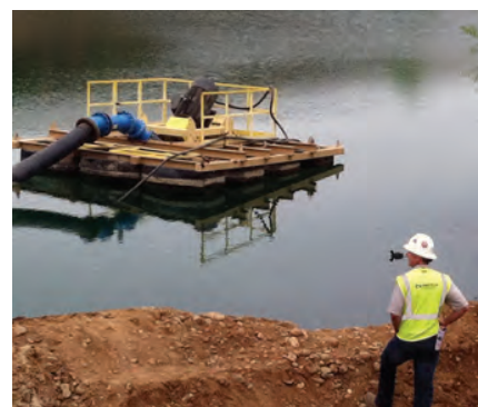
ENGINEER WATCHES AS THE CORNELL PUMP BEGINS START UP
