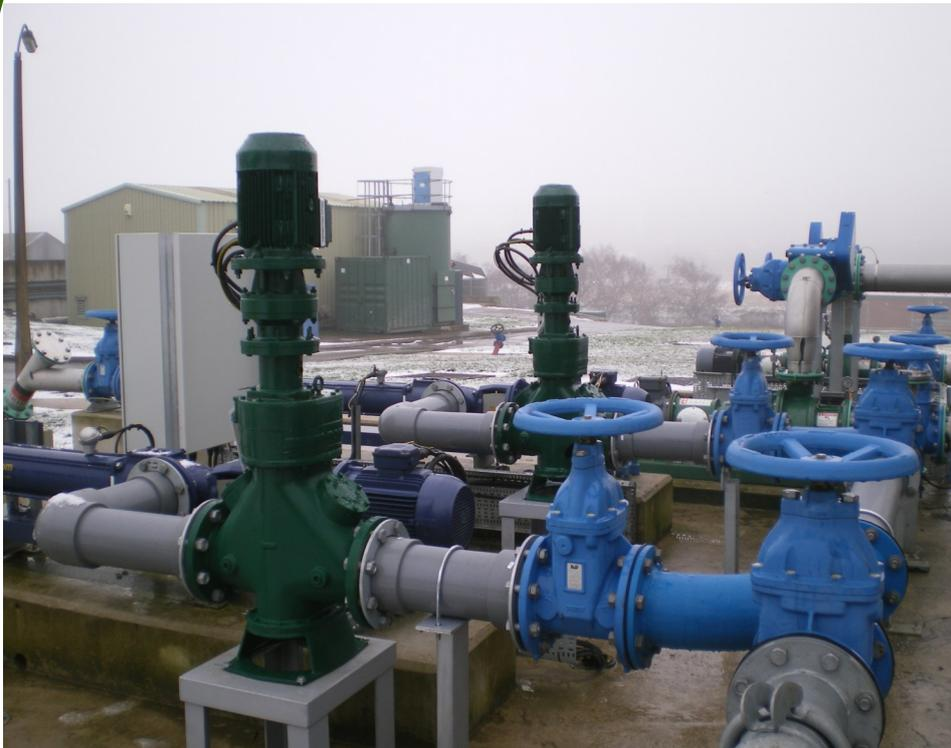
The pump suction inlet was handed to allow a feed from a common line. By turning the pump through 180 degrees and extending the suction pipe work, we ensured independent grinding and pumping. The plant has gone from zero to five grinders within six months due to the success of the initial installation.
