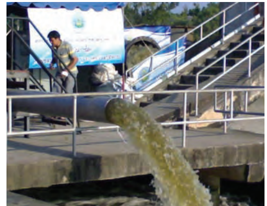
CORNELL'S 14NHG-RP-F18DB DEWATERS MILLIONS OF GALLONS DURING FLOODING
